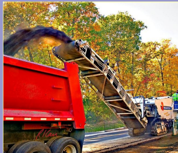
Figure 4: Road being milled:( My construction Photos.)
