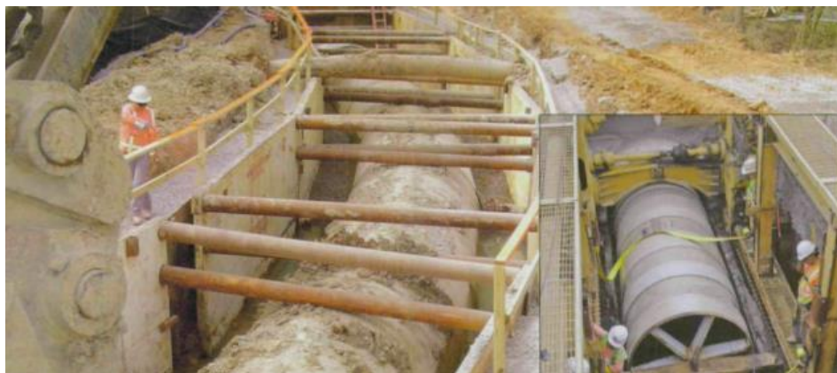
Figure 4: Slip-lining a Curve Source: Sperio, 51
