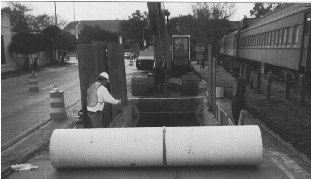
Figure 3: Slip-lining Excavator Source: Lamson, 19
