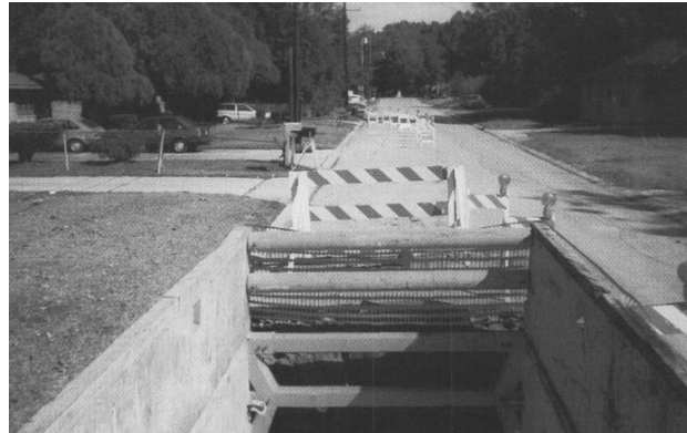
Figure 1: Slip-lining Access Pit
