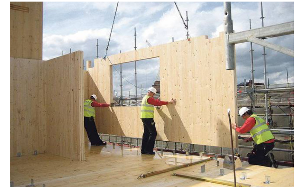
▲ Figure 1 Building Thistleton Waugh CLT Tower in London (Slotover-Smutny)
