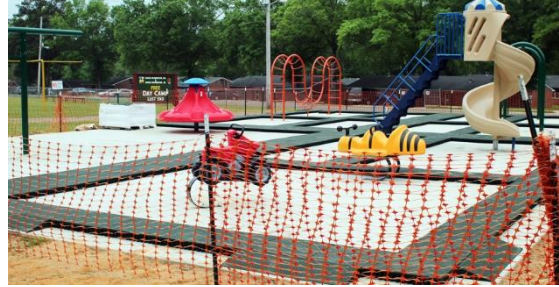
Erected Playground at Greenwood Park with Construction Engineering Technology Students (2015)
