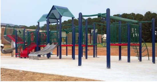
Erected Play System at Glenview Elementary with LA Tech Volunteers (2011)
