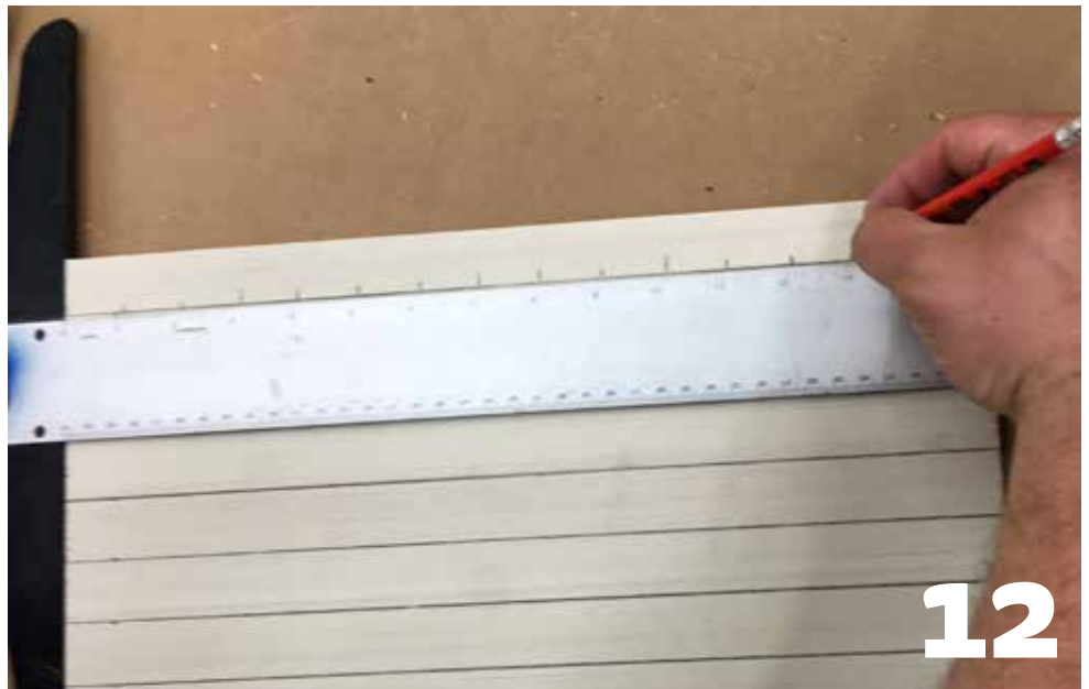
The other plywood panel will be the top of the "Vacuum Box". Use a ruler to draw a 1" grid on it.
