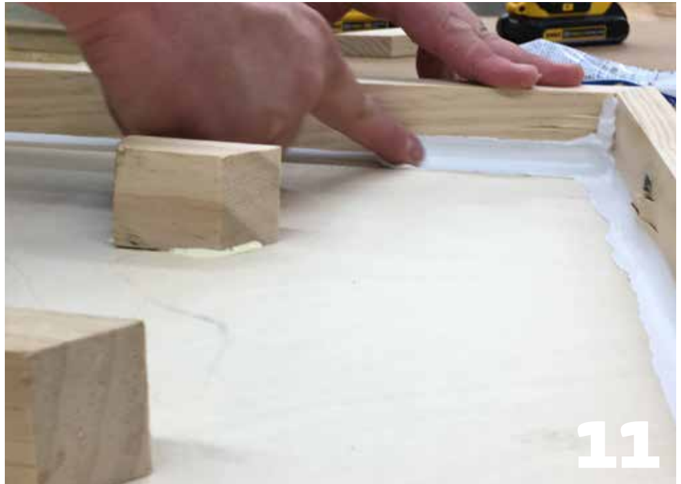
Press caulking into the seams to complete the seal by running your finger along the bead.
